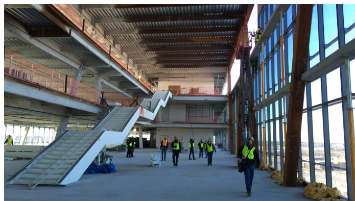
Figure 6. Upper bar atrium with long-span steel staircase connecting levels 9, 10, and 11. Courtesy of Goettsch Partners.
